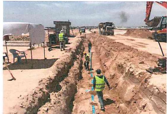
**Backfilled Sand, Laid Macadam Stones and Installed Pipes in Infiltration Basins in June 2018**
