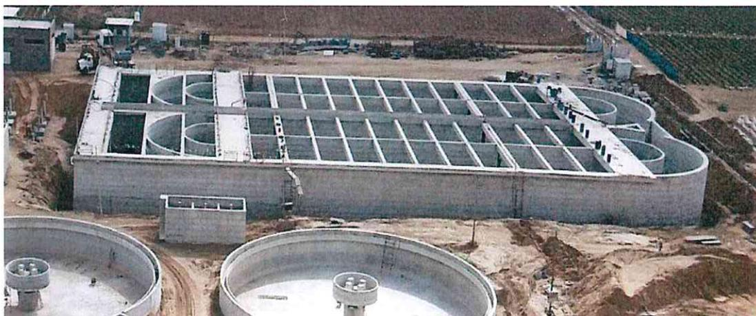
**Casted Reinforced Concrete for the Aeration Tank in June 2018**
