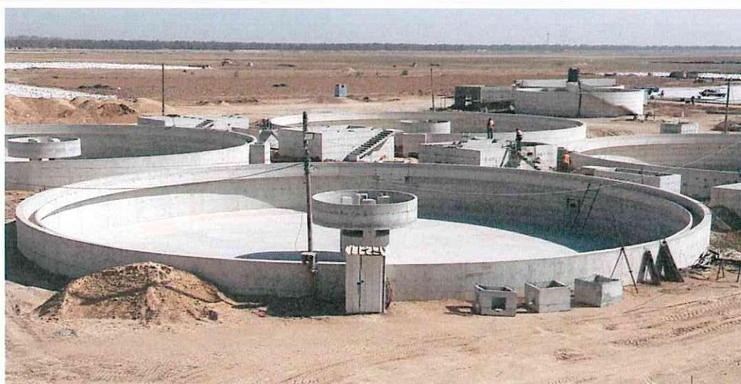
**Casted Reinforced Concrete after Water Tightness Test for the Clarifiers in June 2018**
