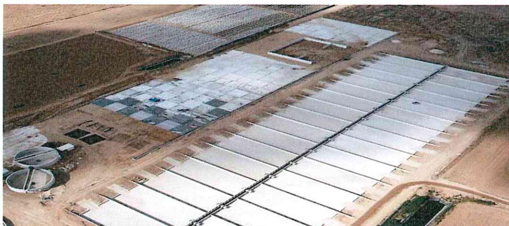
**Casted Reinforced Concrete and Laid Aggregate Layers for Drying Beds in June 2018**
